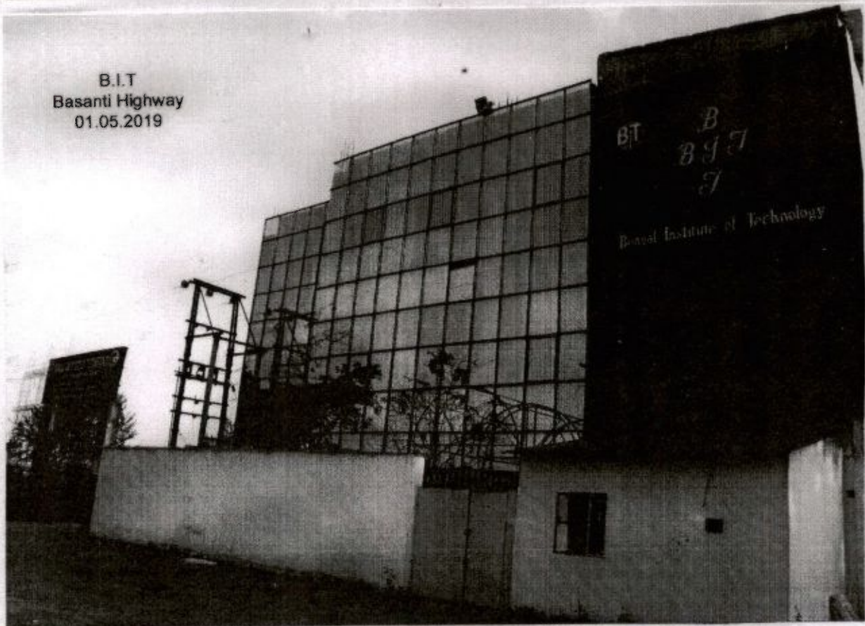
Photographs taken on different dates showing different establishment of business adjacent to Basanti High Way
