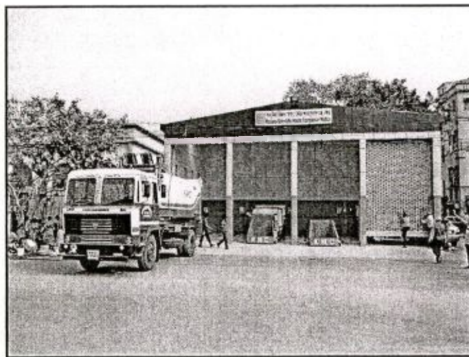
Figure 1.2: Modern scientific waste compactor station at Kalighat park
