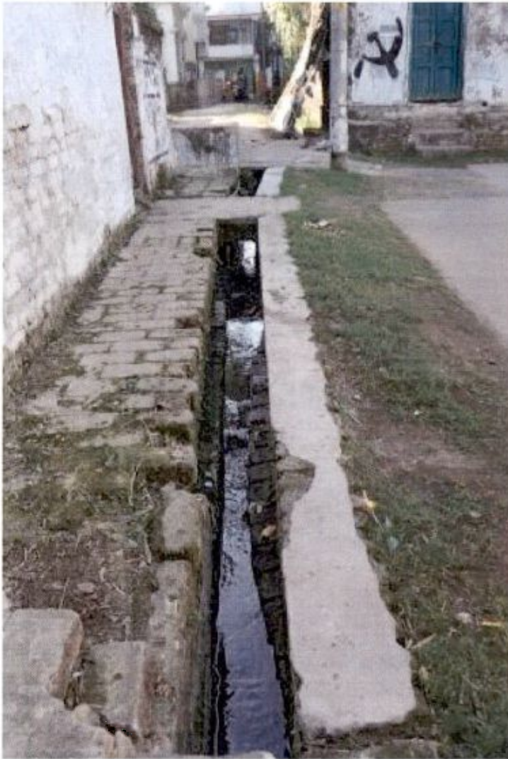
DRAIN OF SIDHWESWARITALA ROAD SLUM
