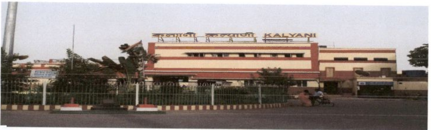
A Sealdah bound train at Kalyani station
