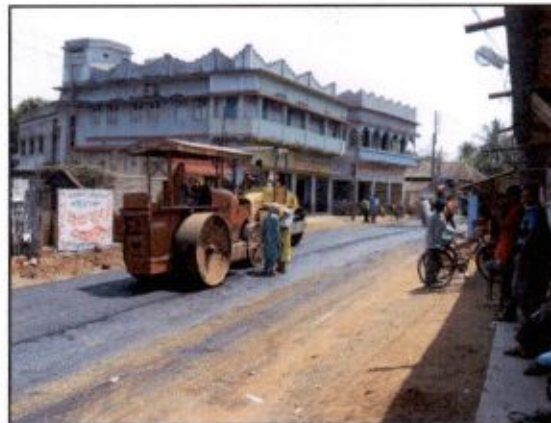
Road Repairing Work Going on
