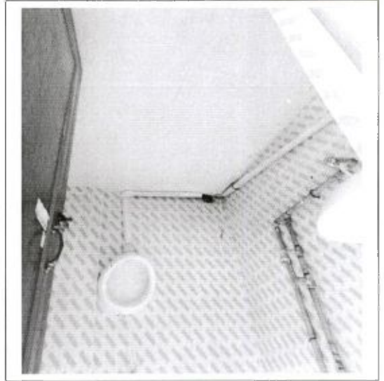
C. Toilet Blocks
