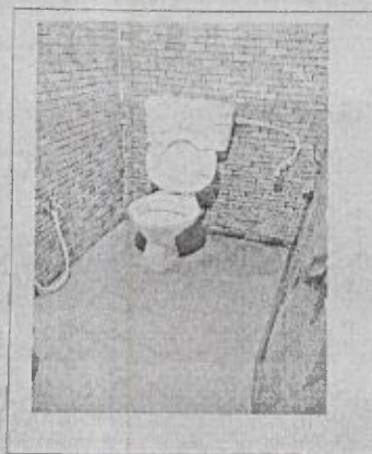
c. Toilet Blocks
