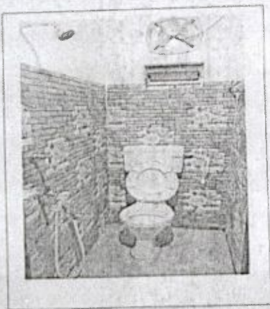
c. Toilet Blocks
